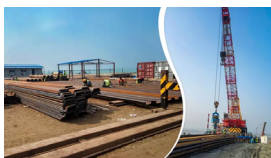
Power Plant Taltoli Jetty Project 2
