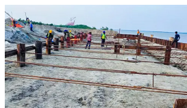
CRCC Jetty Project 1
